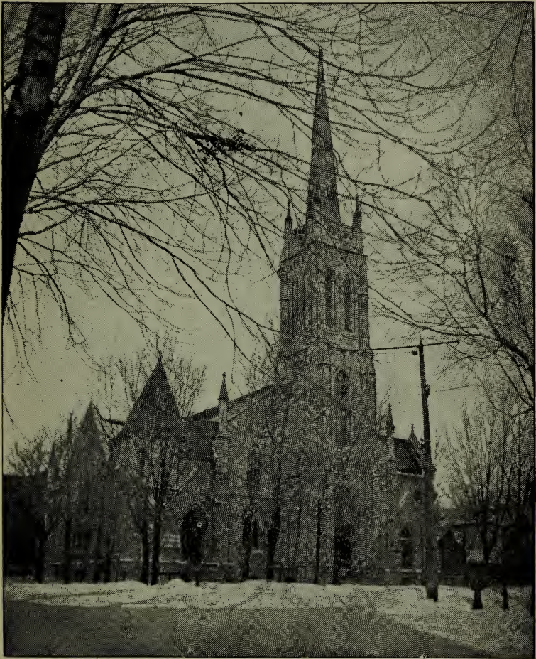
SYDENHAM STREET METHODIST CHURCH, KINGSTON.
